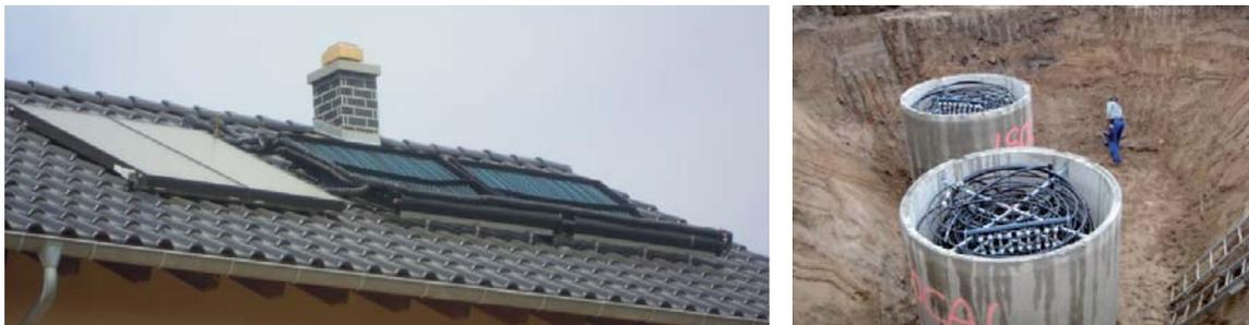
Fig. 3. Solar thermal flat plate collectors (left side of left photo), absorbers (right side of left photo) and ice store (right picture, Source: Isocal)
